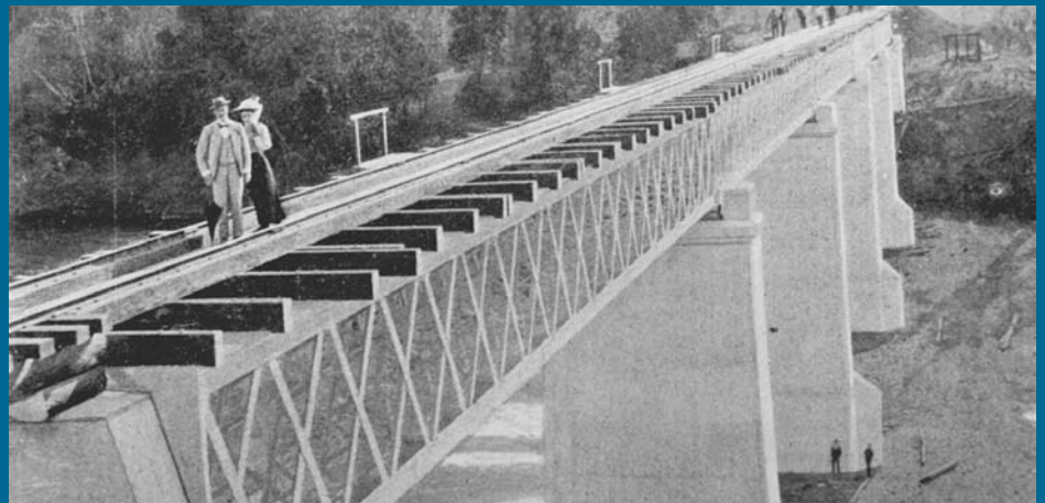
High-level railway bridge at Mirani, ca. 1897.
