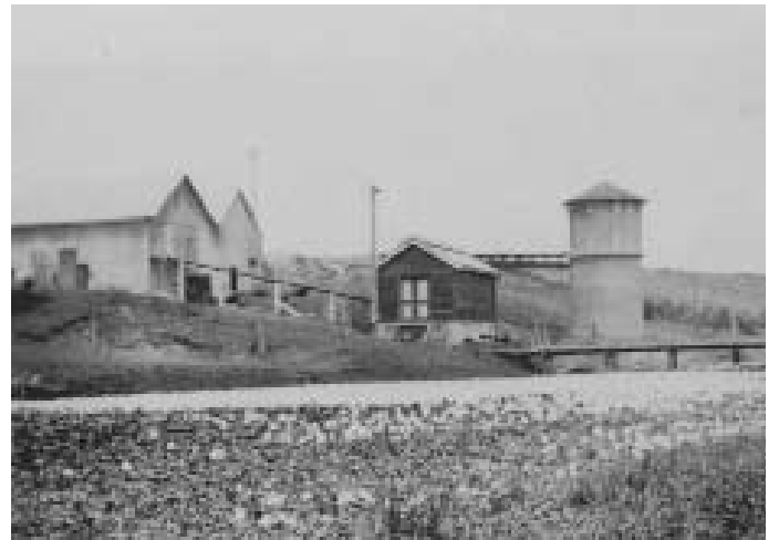
Mackay Water Plant, ca. 1910.
