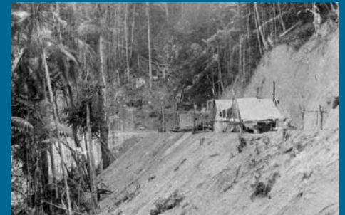
Construction of the road to Eungella, ca 1906-1907.
