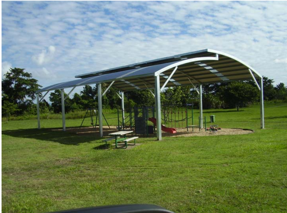
Replacement Shade Structure - Wheeler Drive Park
