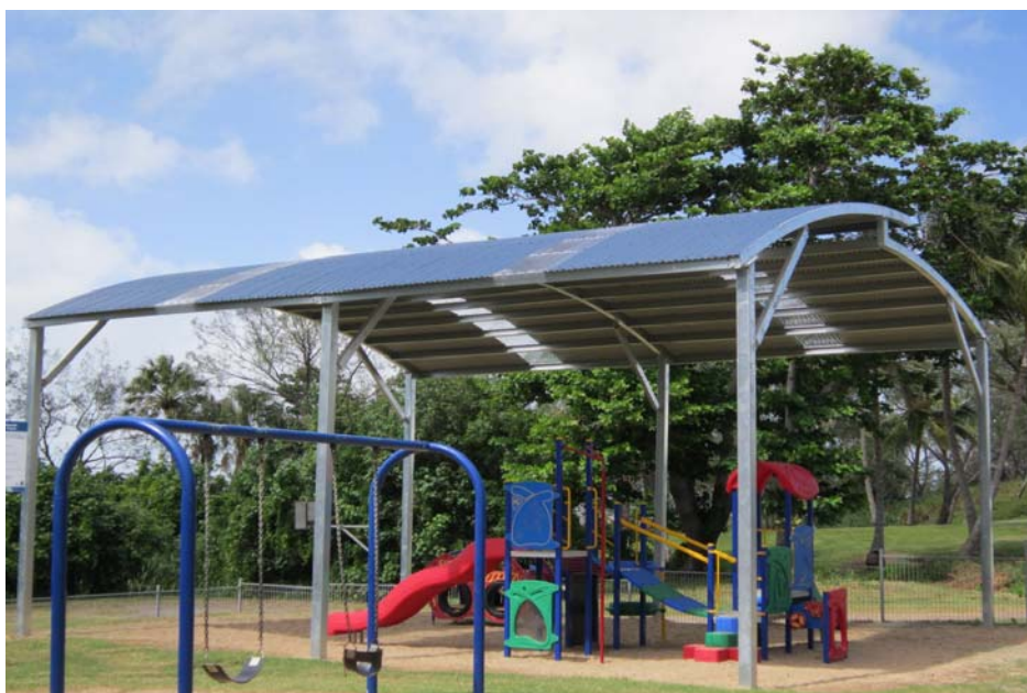
Replacement Shade Structure - Campwin Beach
