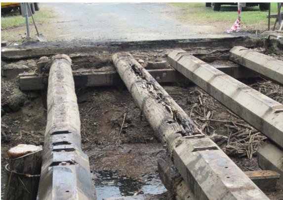
Replace Girder Spans – Lizard Creek
