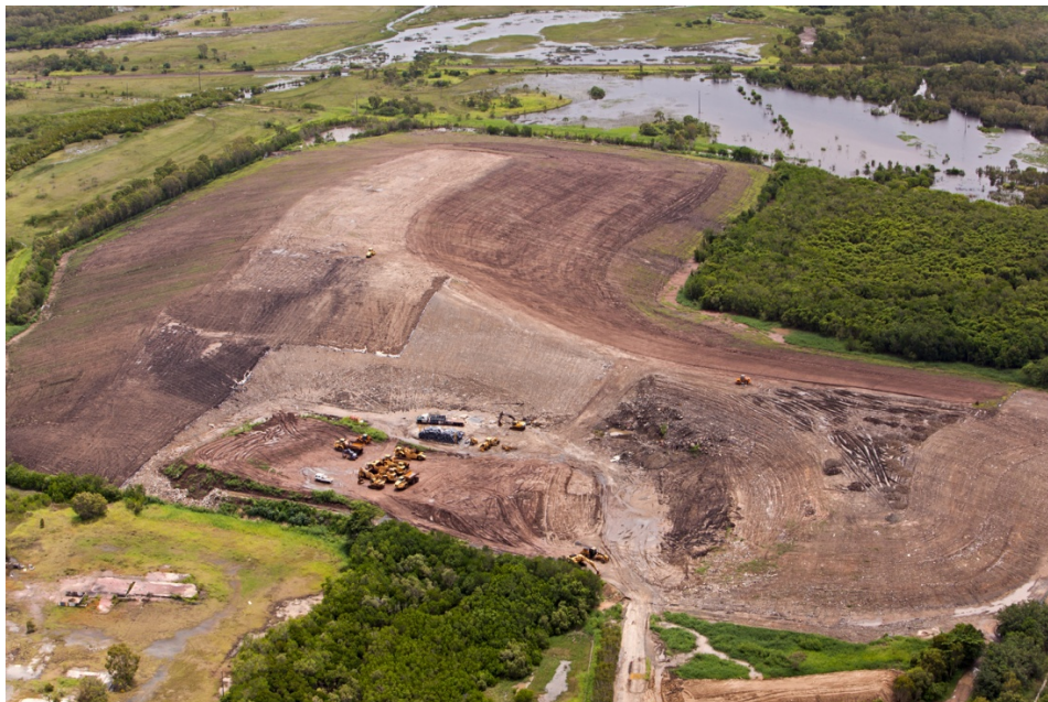
Landfill Bayersville, Capping and Remediation Project
