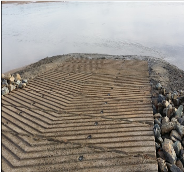
Grasree Beach Boat Ramp – Ramp Units in Place
