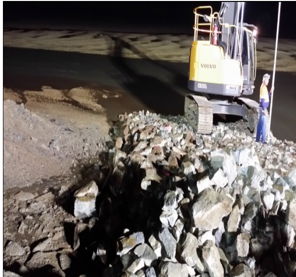
Grasree Beach Boat Ramp – Early Morning Low Tide Foundation Works
