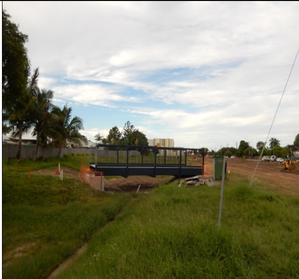
Webberley to Bridge Road – Composite Bridge Structure Across Detention Basin
