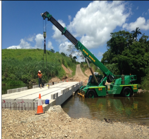
Rostiollas Road – Placement of Deck Units
