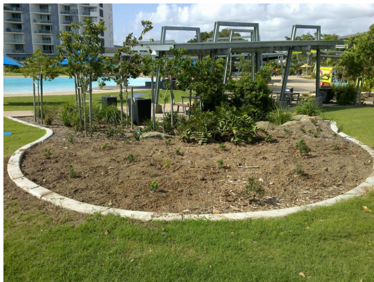
Bluewater Lagoon - Repair of damaged garden and grounds
