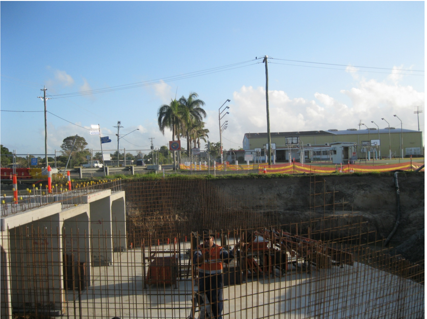
Casey Avenue Culvert Construction
