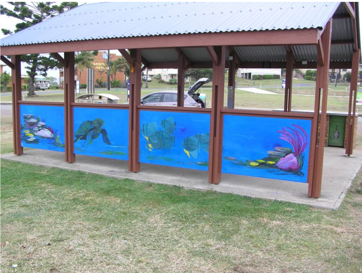
Murals Completed on Second Shelter Sarina Beach
