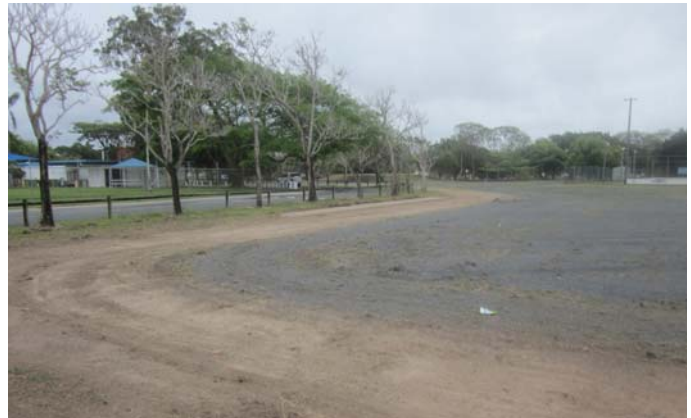
John Breen Park top dressing and drainage work
