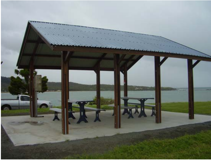
Replacement Picnic Shelter at Coral Point
