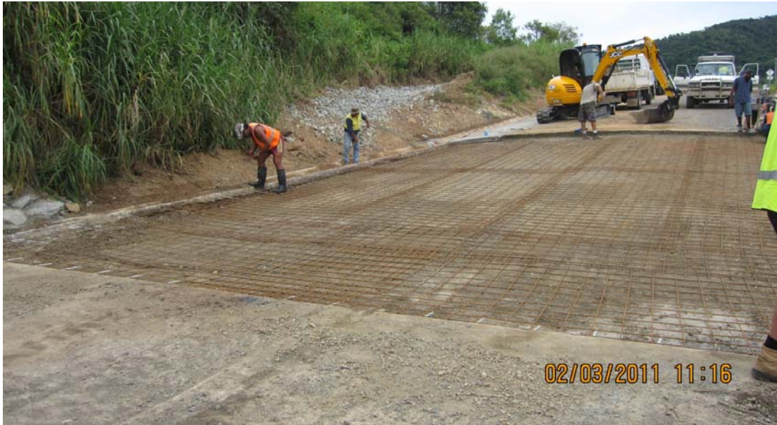
Rifle Range Road Reconstruction – Plane Creek Crossing, repairs after washouts at causeway
