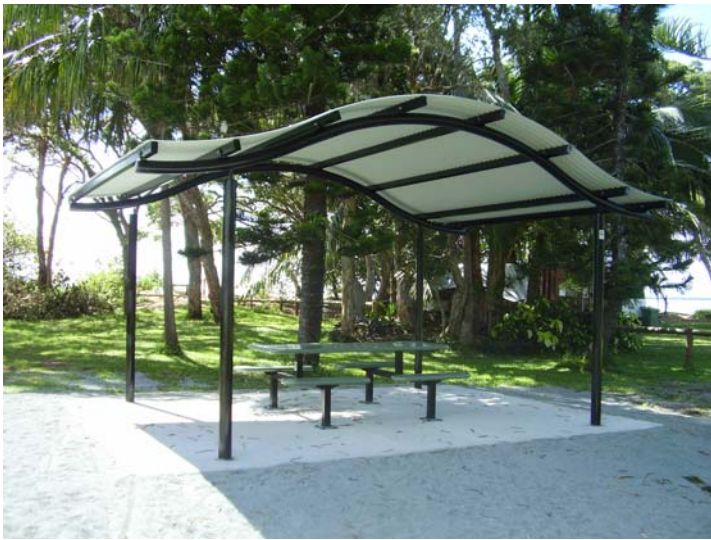
New Picnic Shelter at Melba Park Armstrongs Beach
