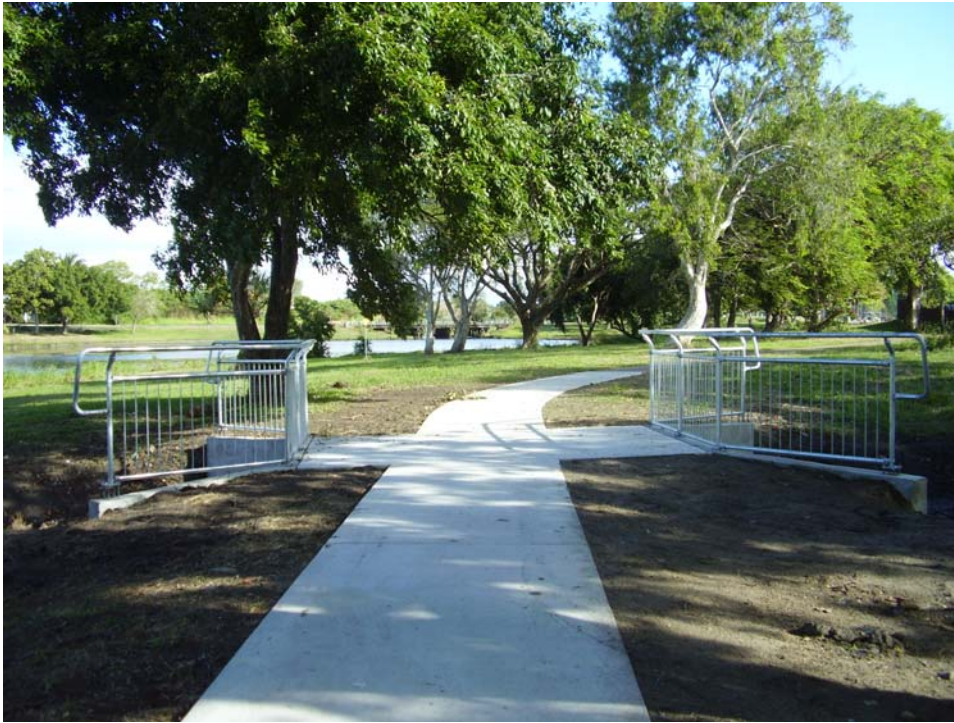
New footbridge Gooseponds
