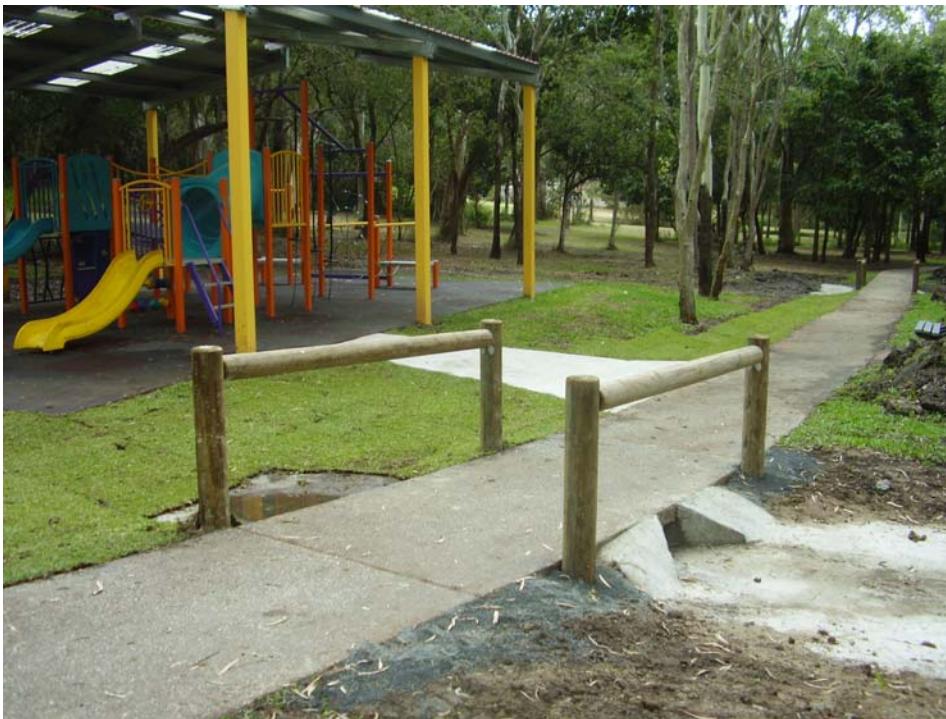
Path and Drainage Work Anniewood Park
