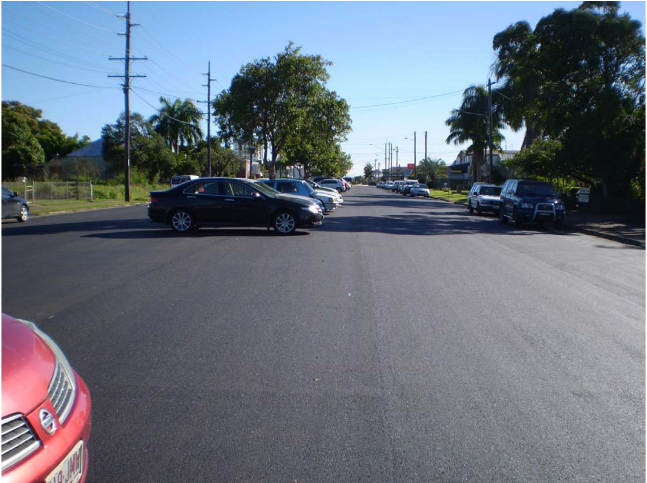
Carlyle Street Resurfacing
