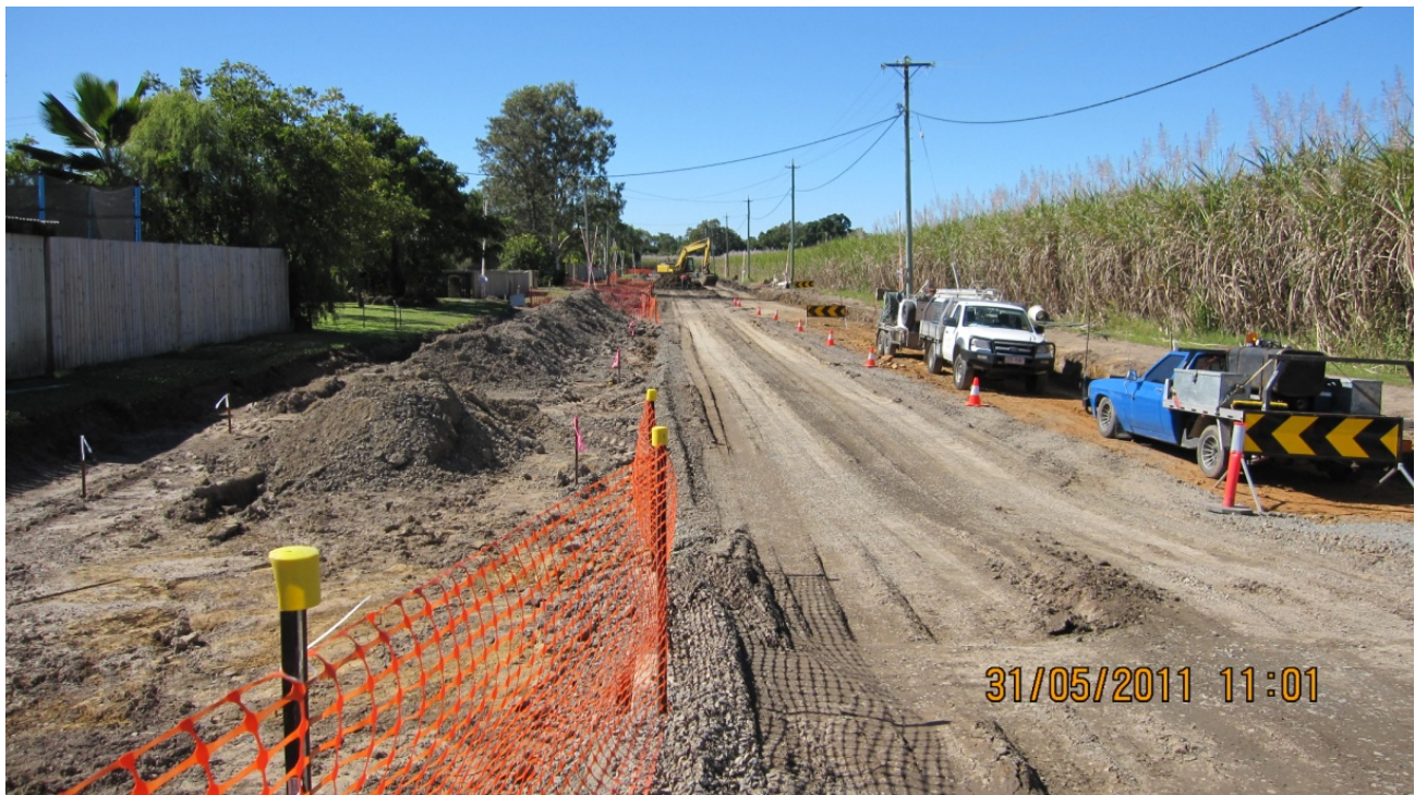
Perry Road Reconstruction, Walkerston
