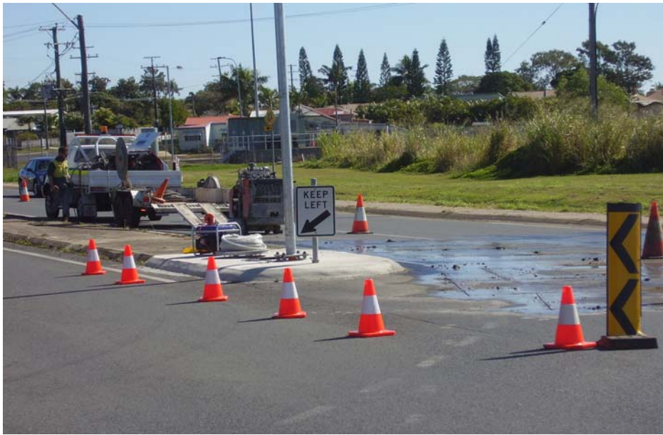
Detector Loop Installation Norris Road Traffic Lights
