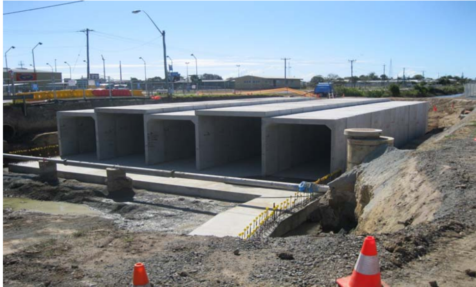
Casey Avenue - Bridge Replacement
