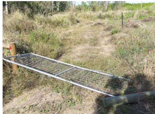
Vandalised fencing and gate at Finlayson’s Point
