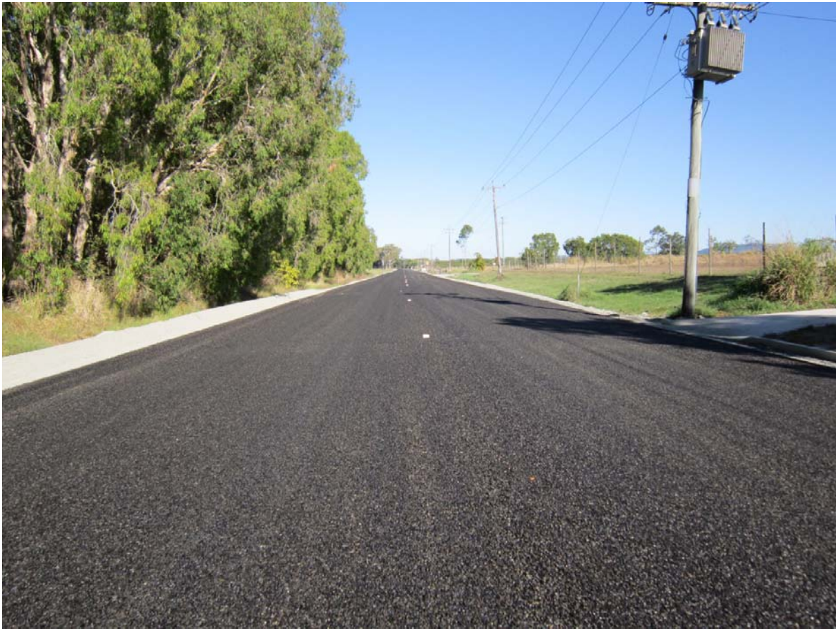
Keeleys Road - Flood Damage Repairs
