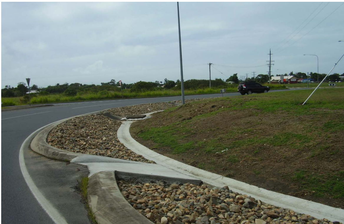
Holts Road Roundabout
