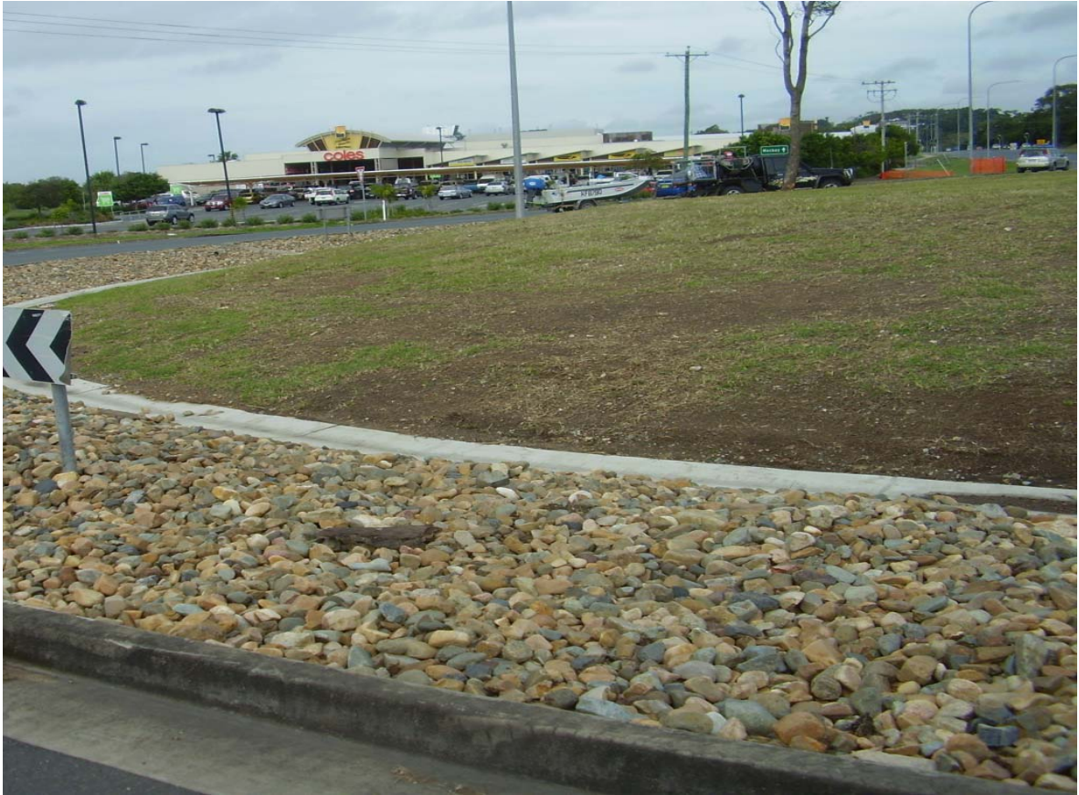
Eimeo Road/ Bucasia Road Roundabout
