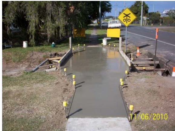
Daly Street, Marian – replace footbridge with box culverts and slab.
