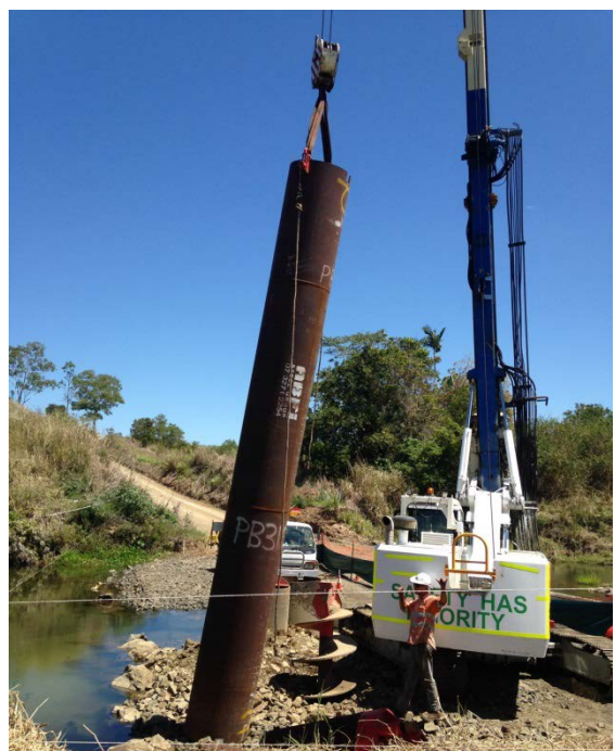
Commencement of Piling works at Murray Creek
