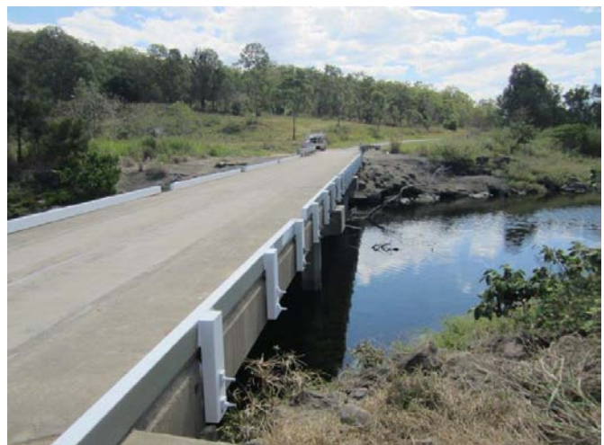
Toon's Bridge Kerb Replacement - AFTER
