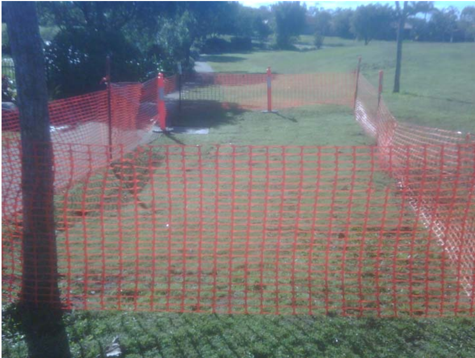
Northview Park Drainage and Turf to Path
