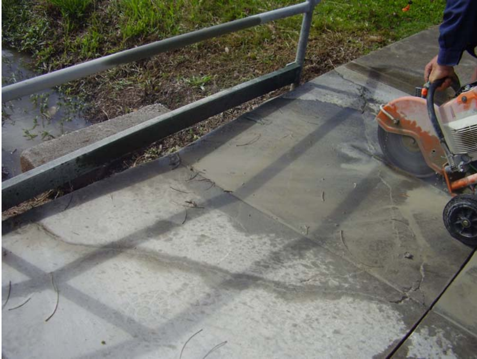
Replacement Culvert and Path- Gooseponds
