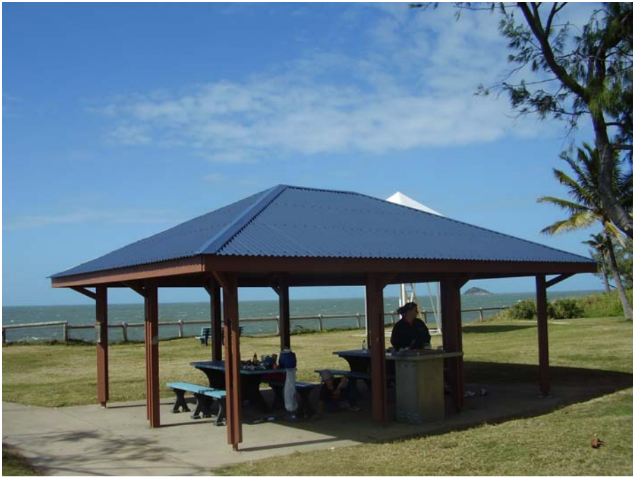
Shelter Roof Replacement - Lamberts Beach 1
