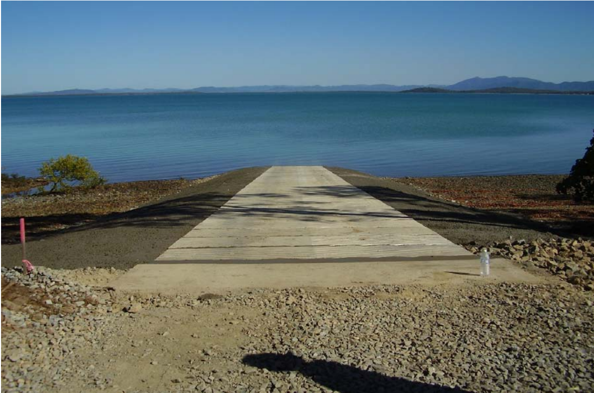
Freshwater Point Boat Ramp
