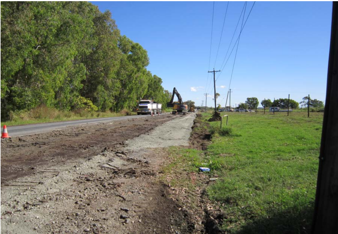
Keeley's Road Flood Damage Repairs
