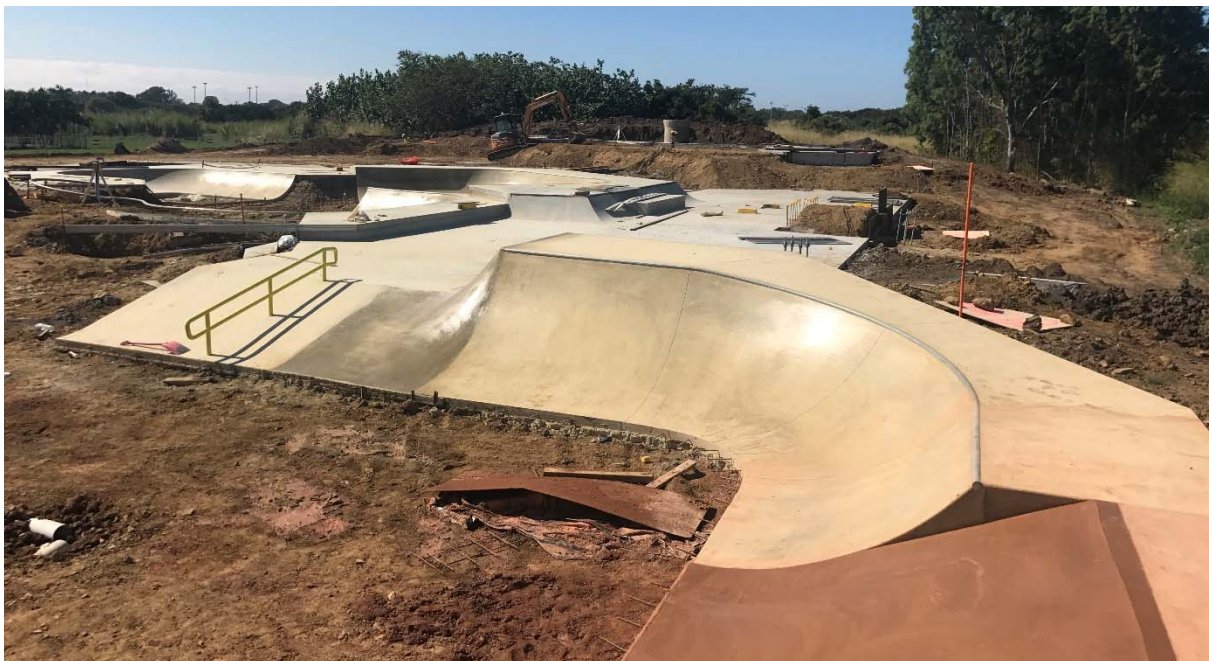
Figure 2 – Street Skate Circuit under construction
