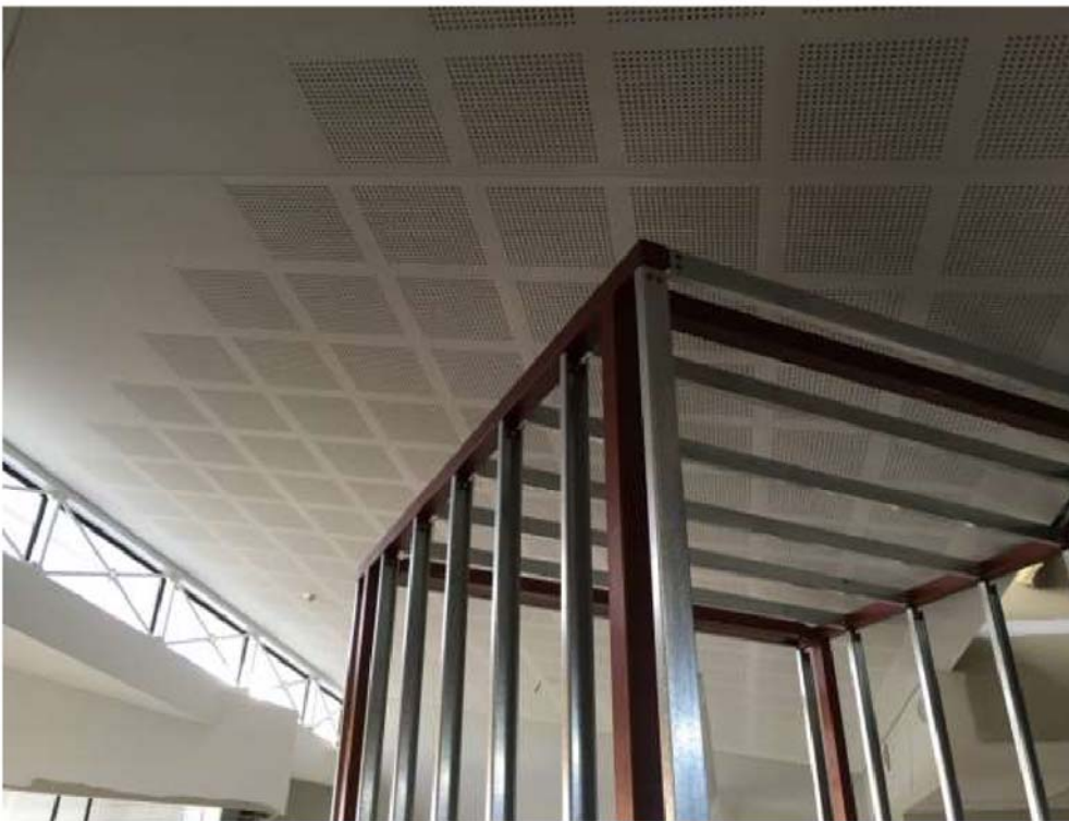
Frame install for elevated reading pod in Children's Area
