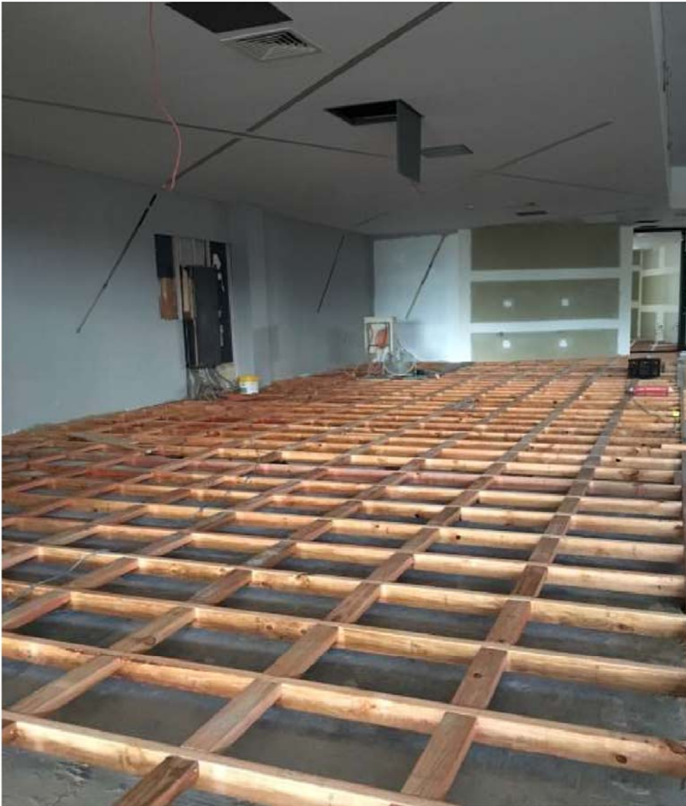
Install floating floor to main collection areas
