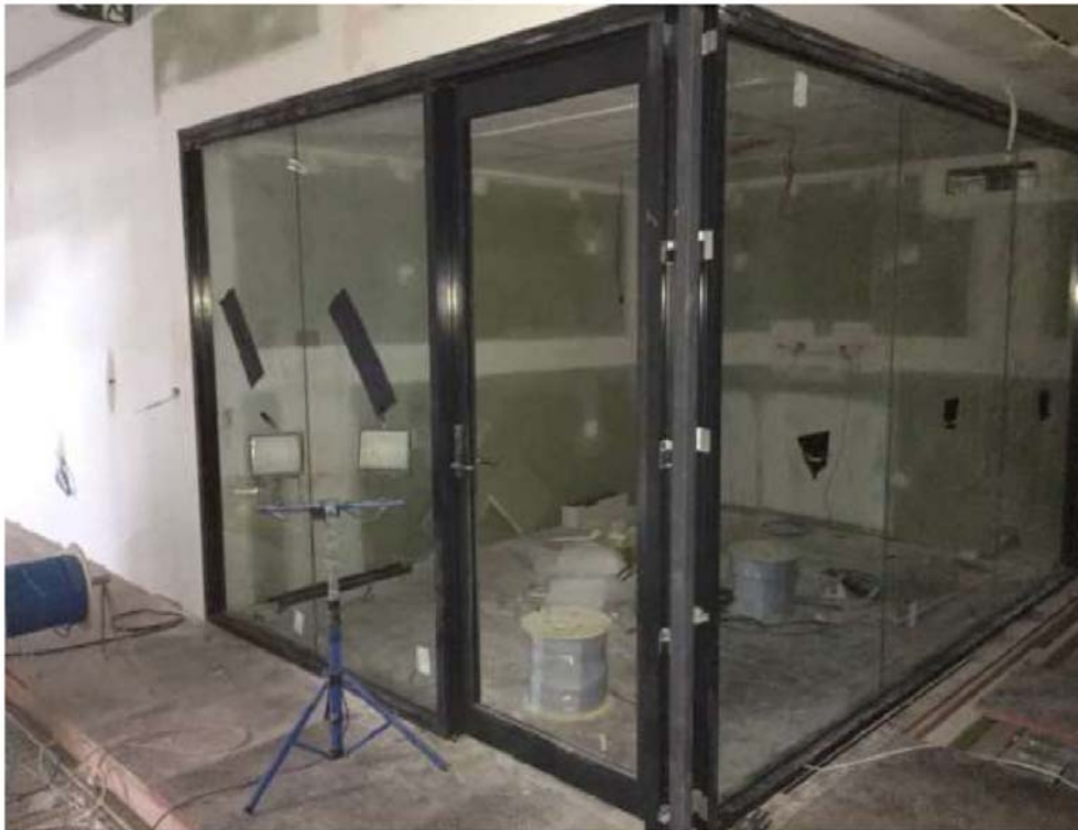
Glazing install to staff meeting room
