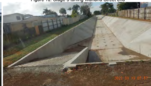
Figure 14: Stage 2 Headwall, ramp complete and turf underway
