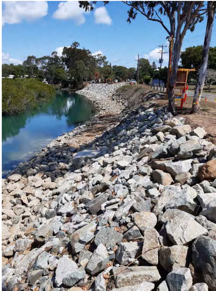
Figure 15: Seaforth Creek Bank Protection Works, from Southern end looking North. Previous Stage 1 works in the middle section where grass has revegetated over the rock work.
