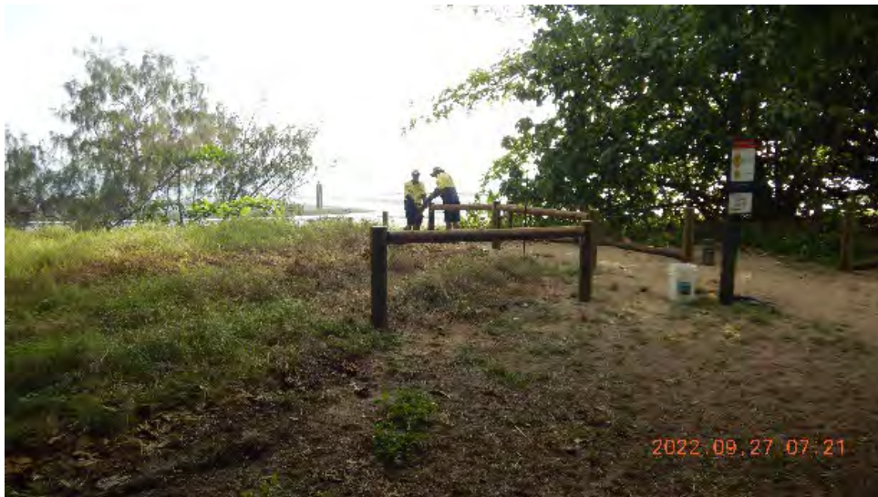
Figure 19: Dune protection post & rail fencing
