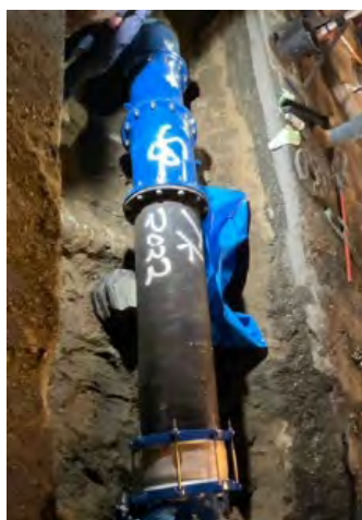
Figure 3: Connection of 375mm water main across Gordon Street
