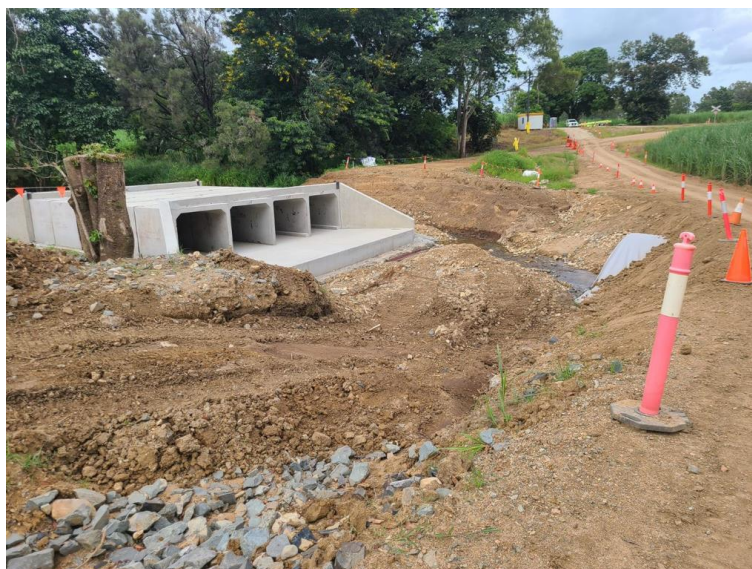
Completion of concrete apron and headwall (51690)
