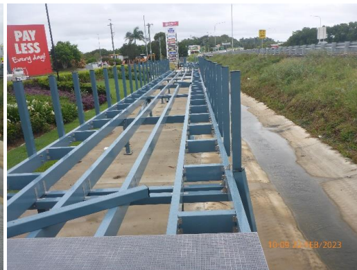
Boardwalk preparation for decking
