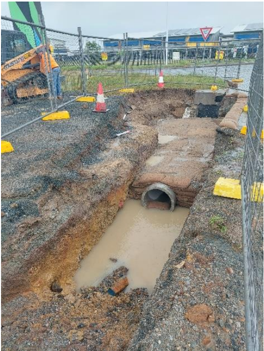
J4 Road Drainage being installed
