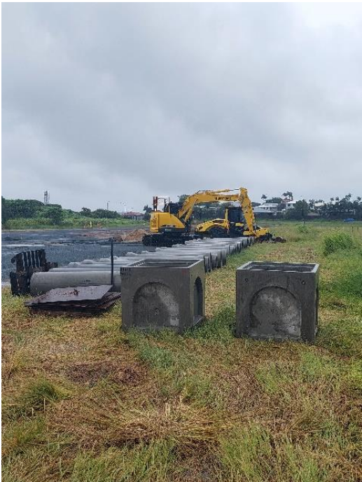
Pipes & pits for drainage
