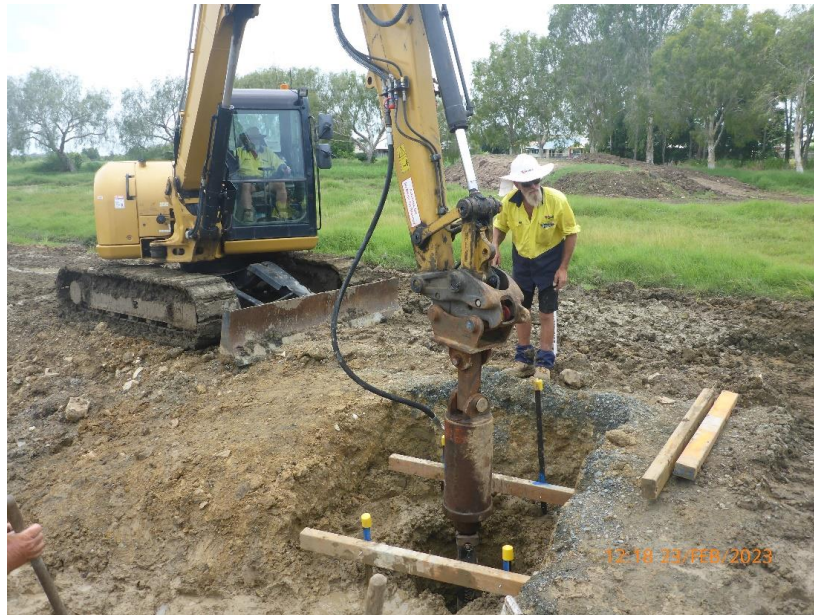
Footing for boardwalk being installed
