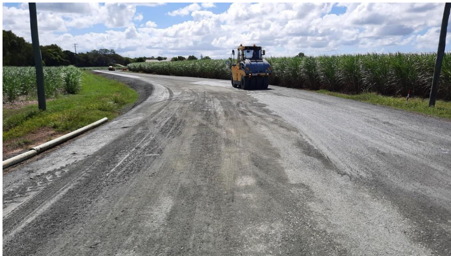
Looking West from Lorne Road direction – Base Pavement Placement
