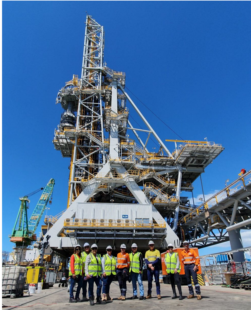
Photo 2: Hay Point Coal Terminal – Ship Loader 2
