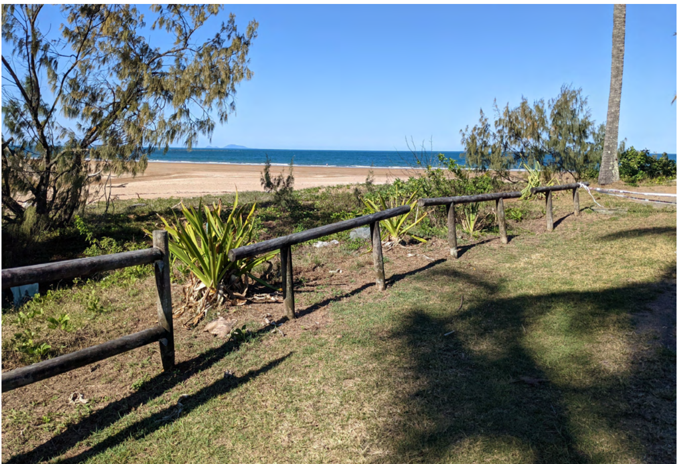
Figure 44: Disjointed fencing around SAR01.
