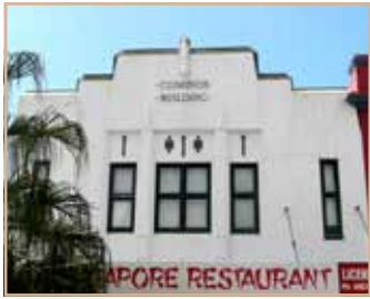
1. Cominos Building 7 Wood St.
