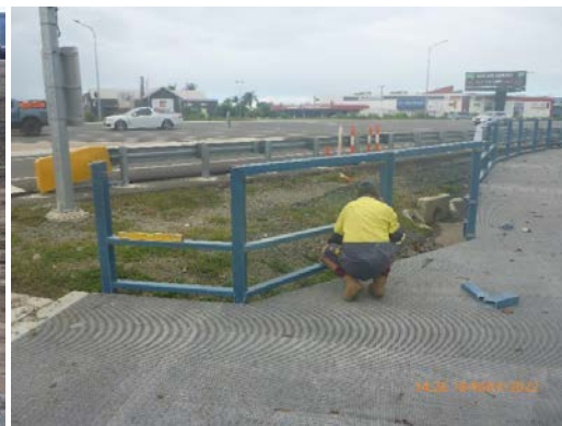
Figure 9: Balustrade installation
