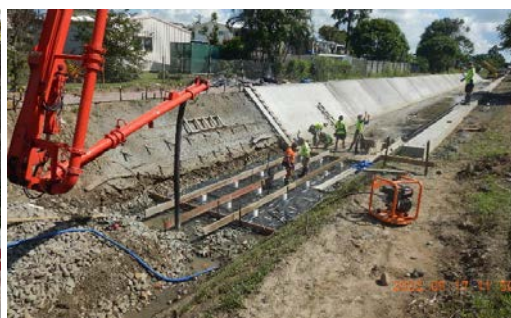
Figure 11: Stage 3 Concrete base
