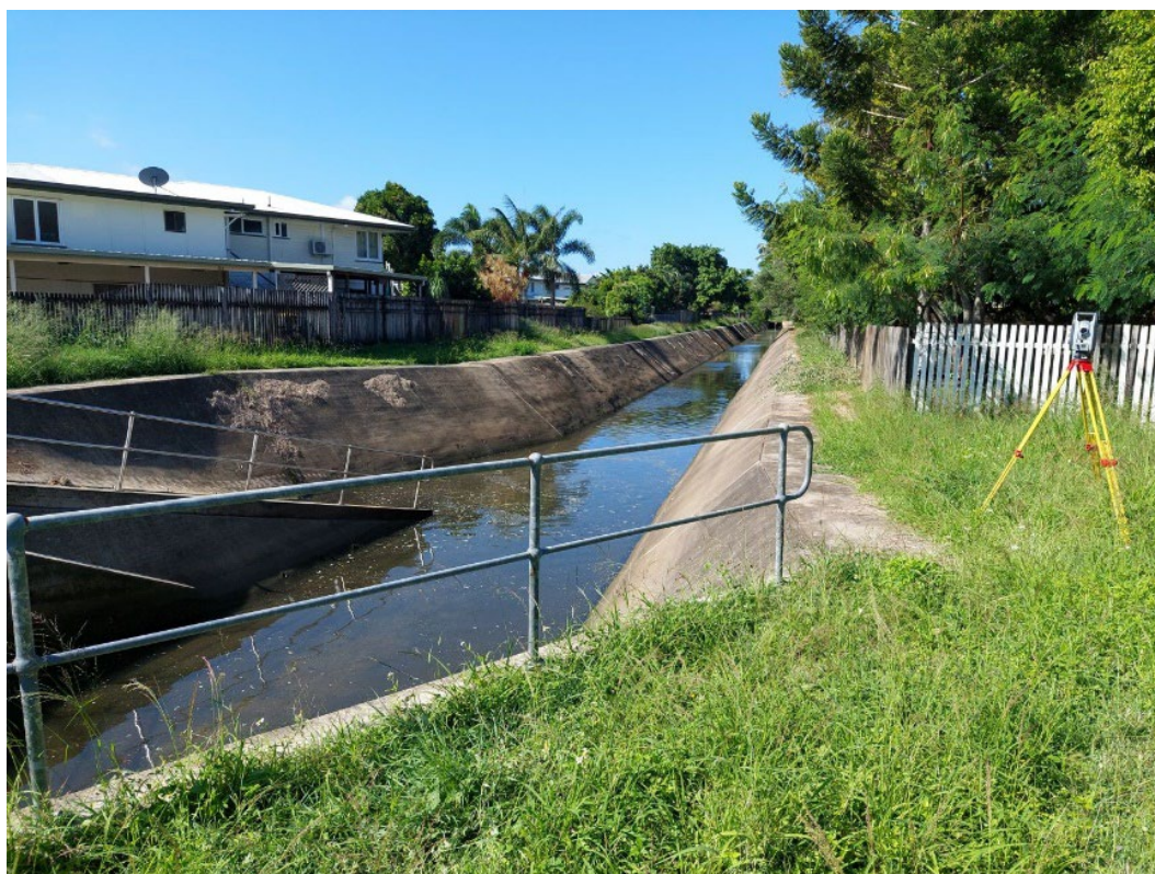
Figure 1: Surveying the Hague St drain for installation of a trash rack
