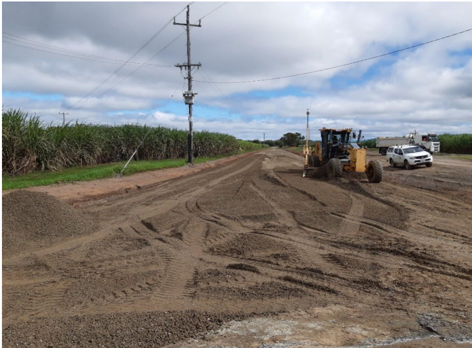
Figure 30: Subbase gravel spreading is underway
