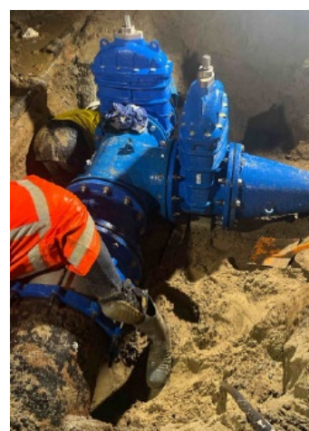
Figure 7: 2 x New 375mm Valves installed
