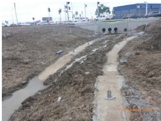
Figure 8: Footing installation
