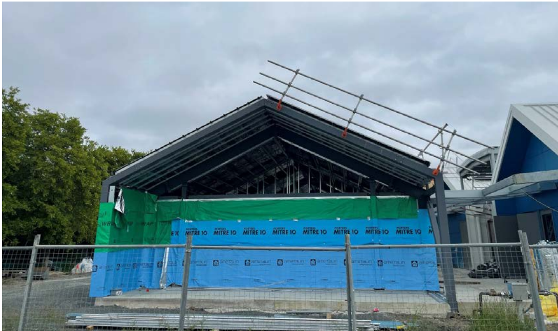
Figure 12: Roof and internal/external wall frames being installed.
