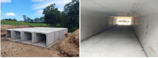
Placement of Culverts Crowns at Owens Creek Loop Road culverts Placement of Culverts Crowns at Owens Creek Loop Road culverts
