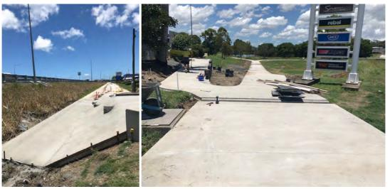
Left: Drain liner and Boardwalk footings. Right: Interconnecting footpaths and retaining wall complete, awaiting the arrival of the bikesafe handrails
