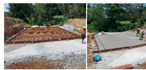
Slab steel reinforcement work at Owens Loop Road culverts
