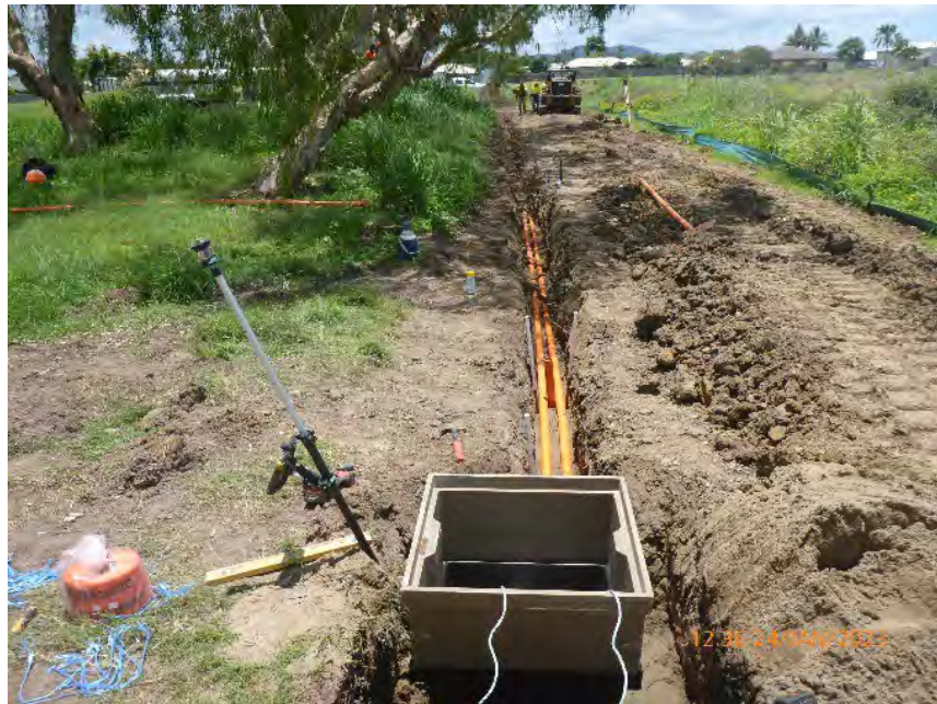
Electrical Conduiting underway
