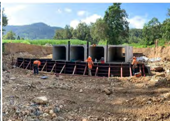
Steel reinforcement work for Apron (51690)
