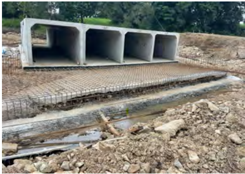
Steel reinforcement re-instatement work for Apron (51690)
