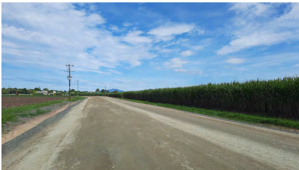
Looking West from Lorne Road direction – Subgrade stabilised.
