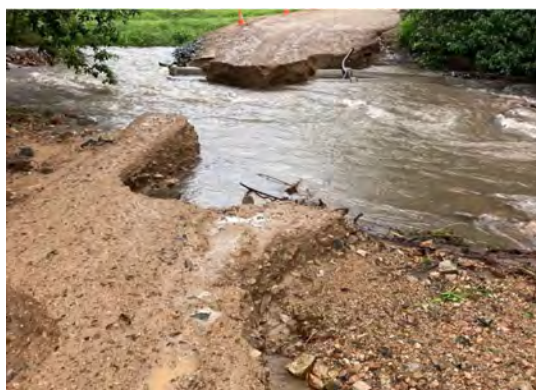
Side Track washout – (51689) at Owens Loop Road culverts
