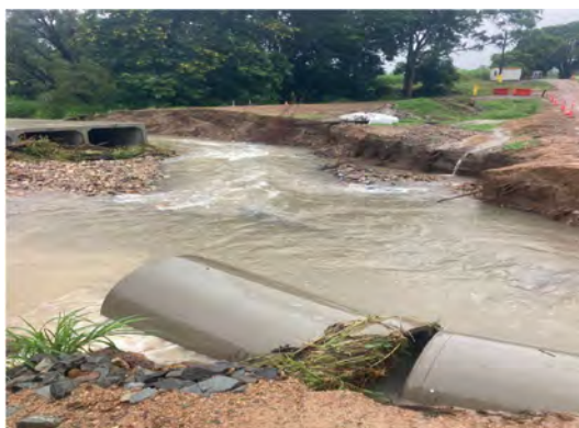
Side Track washout – (51690) at Owens Loop Road culverts
