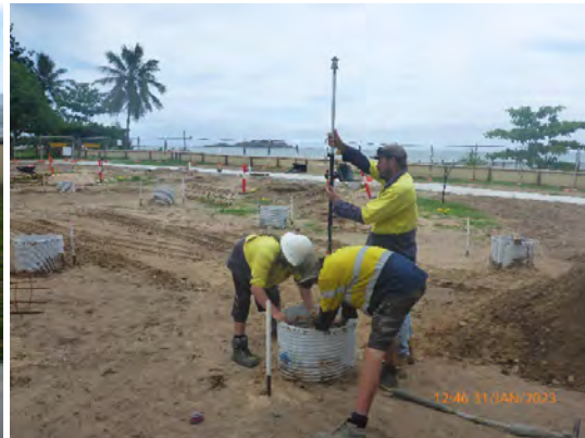
Piers for shelters being installed
