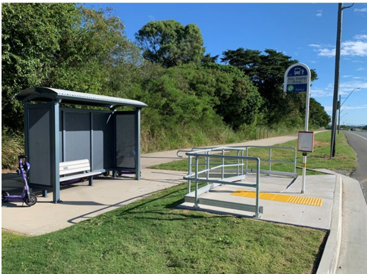
Ron Searle Drive completed bus shelter
