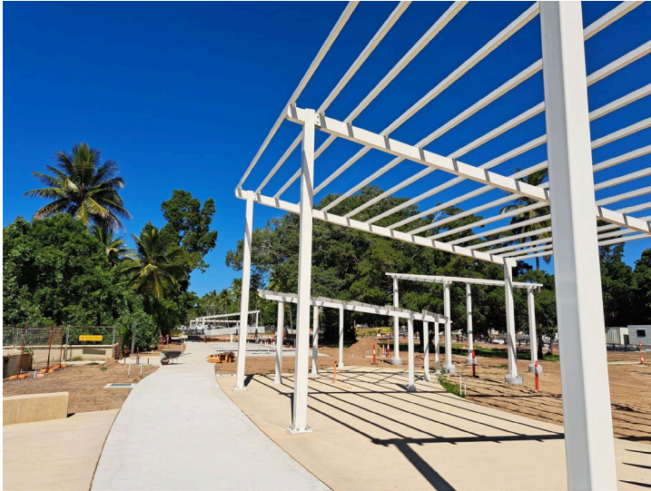
Seaforth Esplanade redevelopment construction progress
