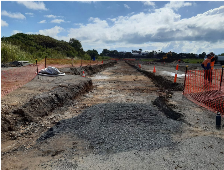
Northern Beaches Community Hub road construction
