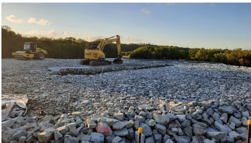
Figure 30: Southern carpark rock placement almost completed; pipe bedding completed for RCP installation.
