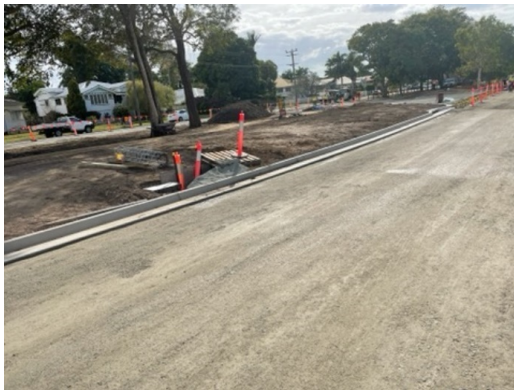
Figure 21: George Street final pavement layer
