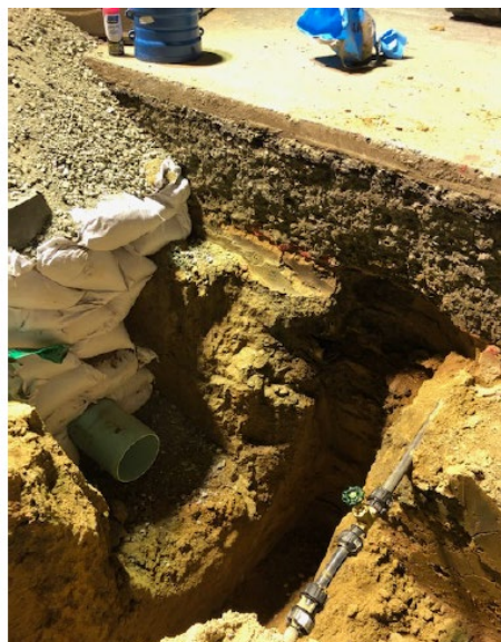
Figure 10: Preparation for new thrust block
