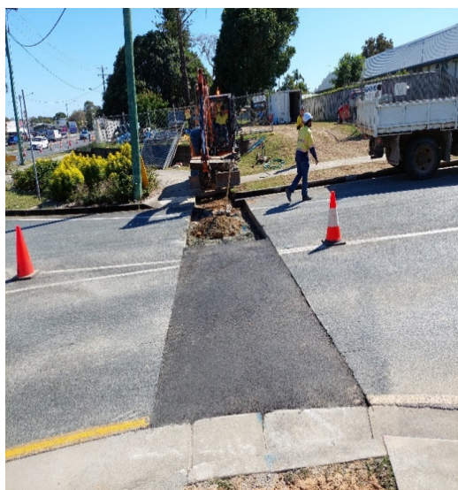
Figure 17: Coles St road cutting
