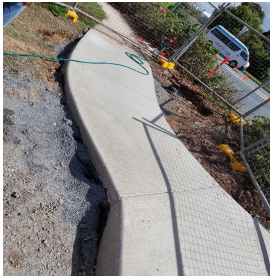
Figure 18: Reinstatement of the concrete foot path (Cole's round about)
