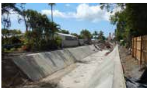
Figure 10: Concrete base, batters and cut-off walls
