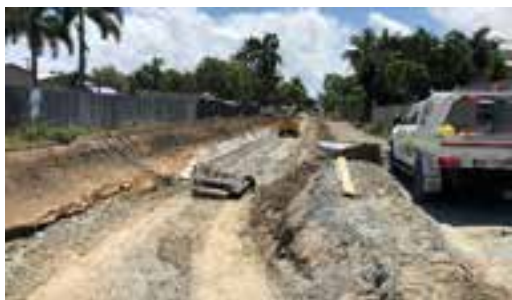
Figure 9: Stage 3 rock base installed
