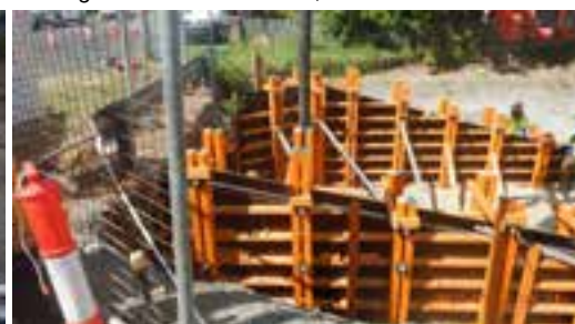
Figure 12: Concrete base, batters and cut-off walls
