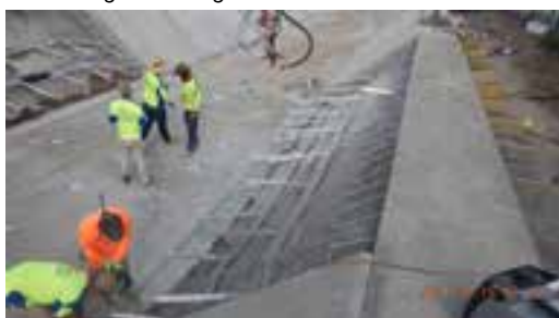
Figure 11: Stage 3 rock base installed
