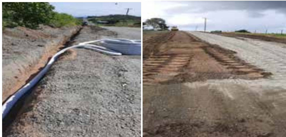
Figures 22 & 23: Sub-soil Drainage & Stabilisation is completed in final section on Glenella Richmond Road
