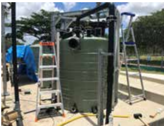
Figure 4: Agitator installation
