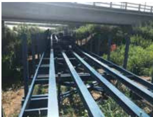
Figure 7: Ongoing Composite Boardwalk installation
