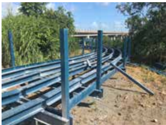
Figure 7: Ongoing Composite Boardwalk installation
