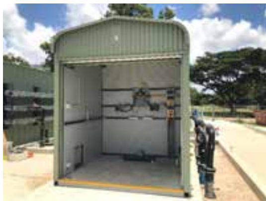
Figure 3: Chlorine dosing shed installation.
