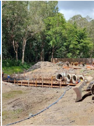
Headwall construction underway
