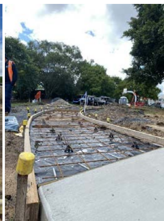
Concrete Footpath Formwork
