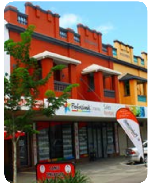
Andrews Treasure Store, 2016, Mackay Regional Council Note that the upper-level 'Andrews' signage has been removed
