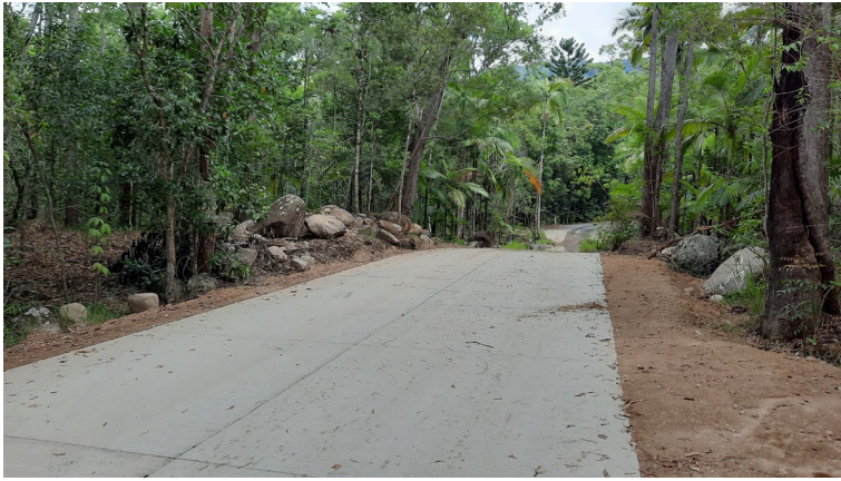
Gorge Road Concrete Pavement
