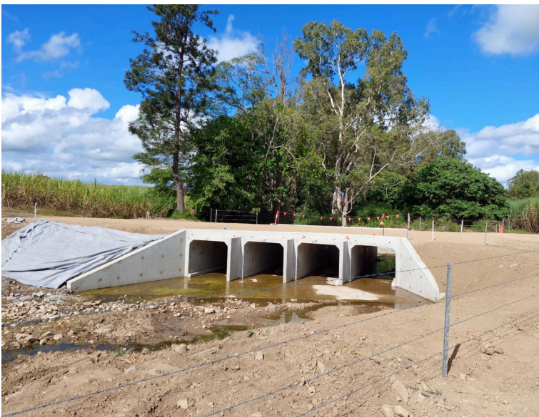
Culvert Replacement nearing completion
