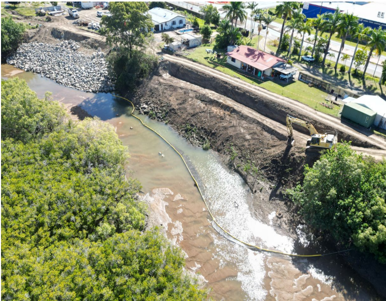
Rock Bank Protection Works
