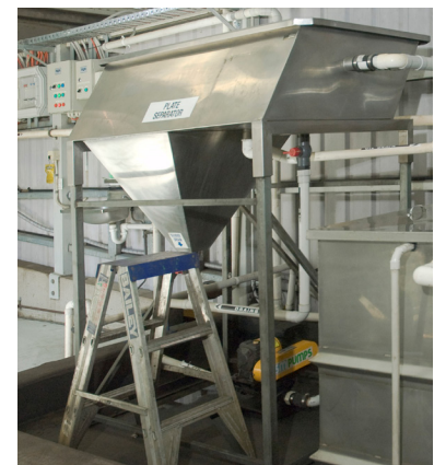
A bank of individual 2,000 litre capacity grease arrestors and a typical oily water separator.
