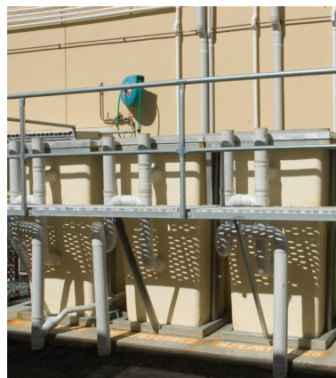
A bank of individual 2,000 litre capacity grease arrestors and a typical oily water separator.
