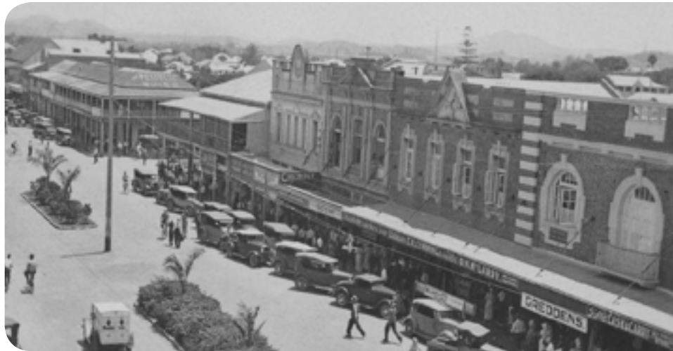
North Side of Victoria Street ca. 1930, looking west from Marsh and Webster, from the right Dalrymple building, then Dalrymple number two, then Armati Pharmacy showing 'Chemist' in the awning, and lastly Hamilton's building.
