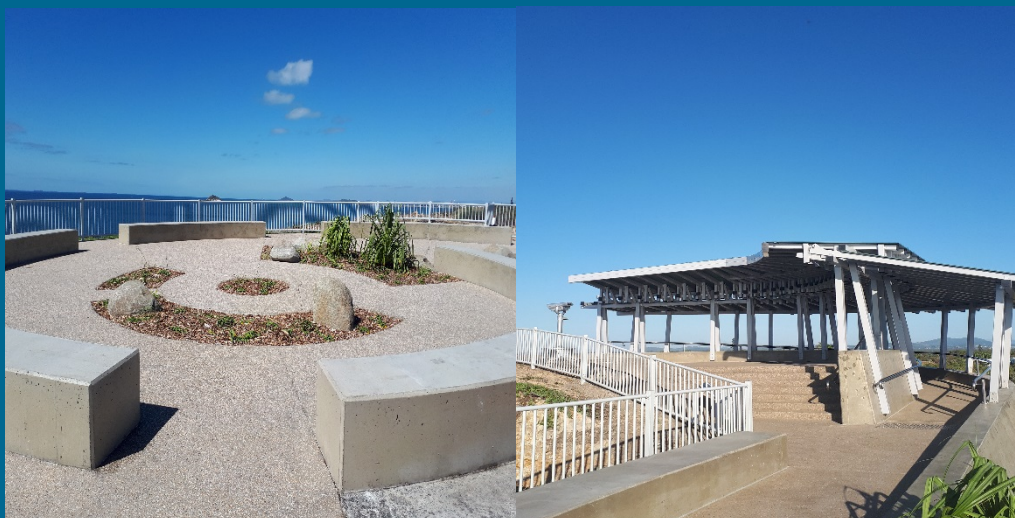
Whale Watching Pavilion at Lamberts Beach Lookout, officially opened on August 18.
