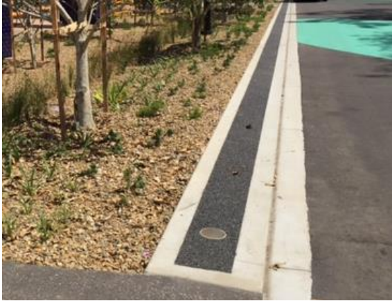
FIGURE 10. PRE-TREATMENT OF SURFACE RUNOFF PRIOR TO DISCHARGE TO WICKING ZONE.
