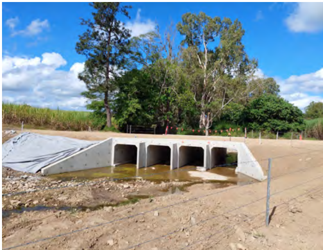
Culvert Replacement nearing completion
