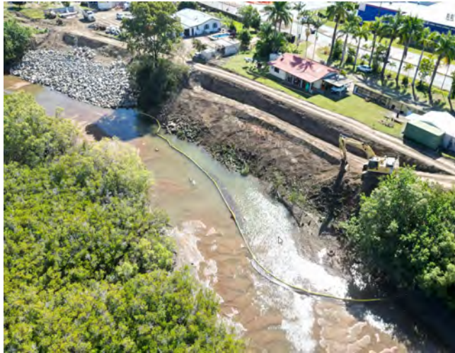
Rock Bank Protection Works
