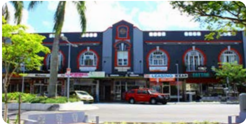
Dalrymple Building, 2016, Mackay Regional Council
