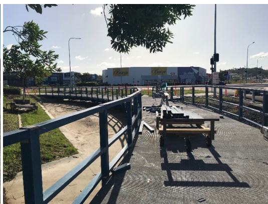
Figure 8: Balustrade installation
