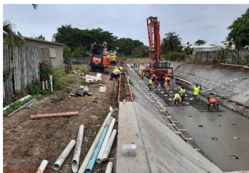
Figure 10: Stage 3 Concrete base and Rate Wall
