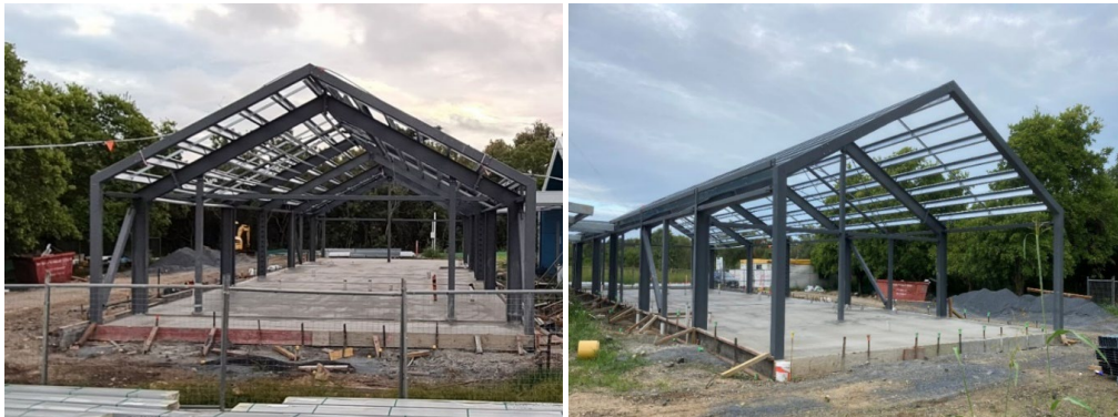
Figures 15 & 16: Building Slab Complete and Structural Steel Erected - Stage 2
