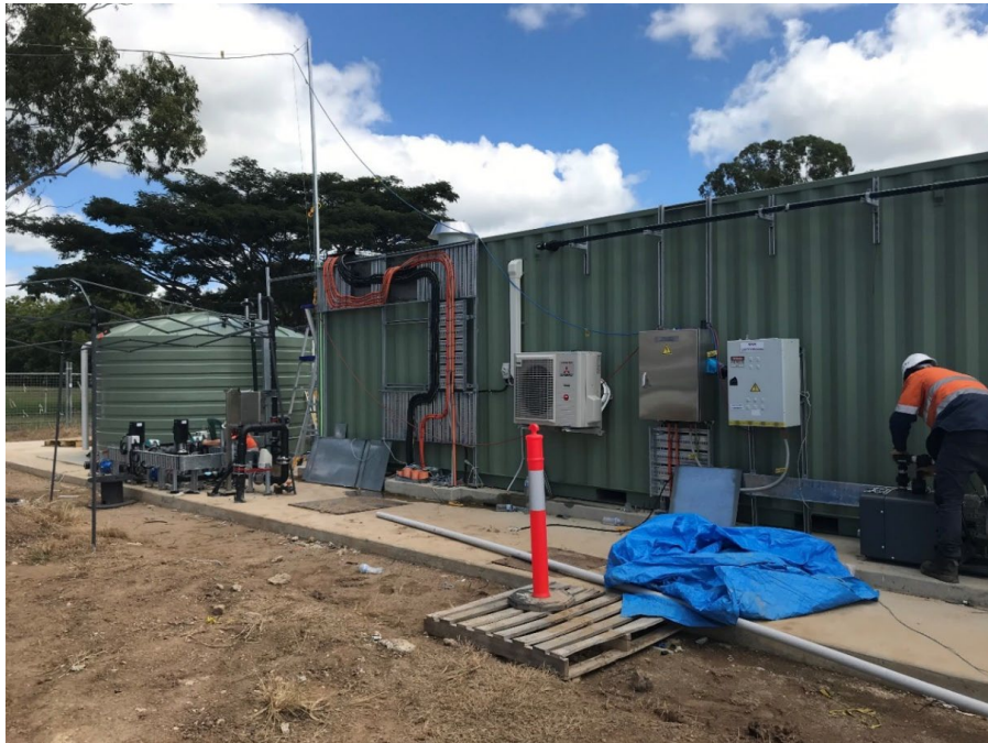
Figure 2: package plant container - electrical cable trays and external equipment
