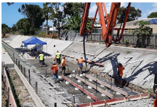
Figure 9: Stage 3 Concrete Base
