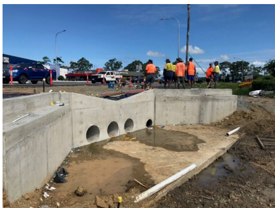
Figure 7: Headwall and abutment (stripped)
