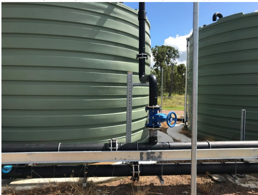
Figure 3: Ground water storage tanks and external pipe work
