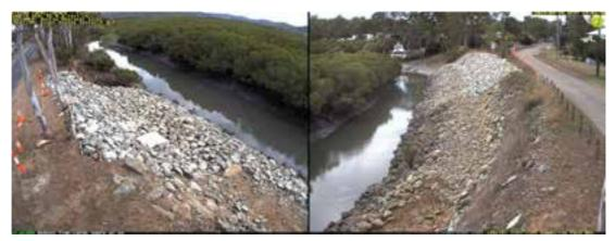
Figure 11: Seaforth Creek Bank Protection Works, from Southern end of existing rock protection looking North on the right, looking South on the left. Previous Stage 1 works evident where grass has revegetated over the rock work.
