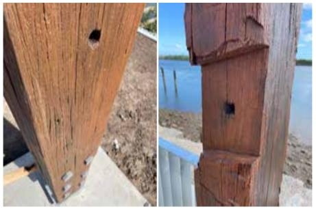
Figure 16c: Salvaged 1895 timber used on new structures
