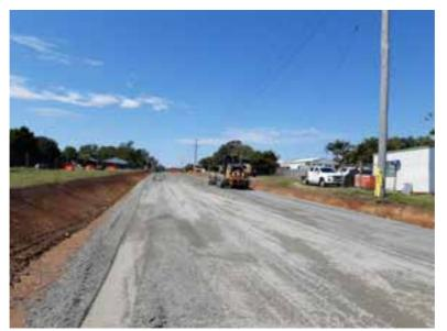
Figure 20: Subbase layer - Looking South from railway toward Roundabout
