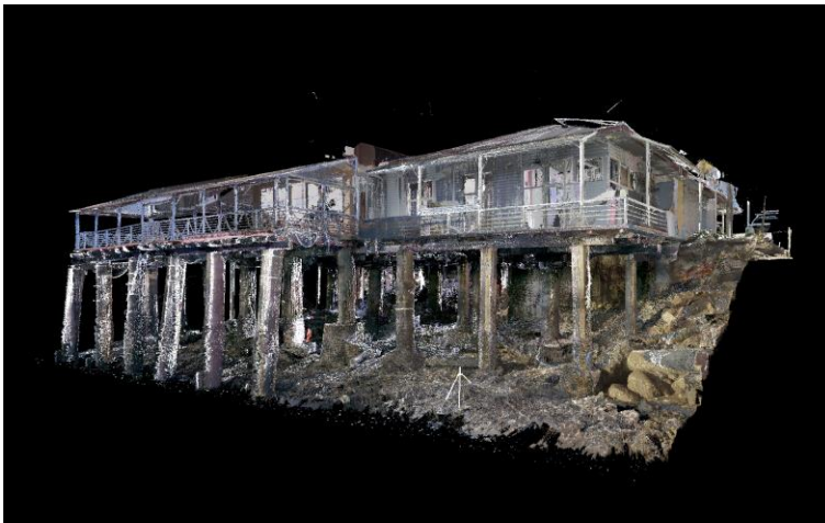
3D Point Cloud of 8 River St Piers
