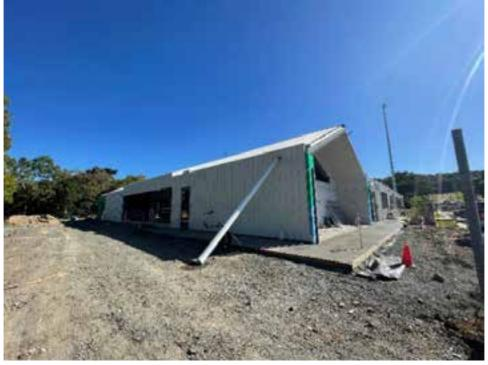
Figure 14: Installation of external wall cladding
