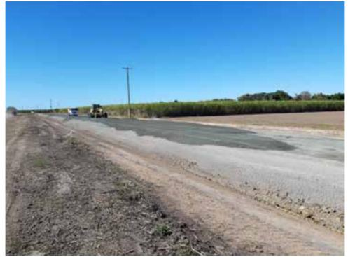
Figure 26: Base gravel spreading is underway
