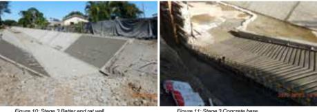
Figure 10: Stage 3 Batter and rat wall
