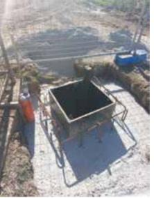
Figure 3: Bore Site: new electrical pit construction
