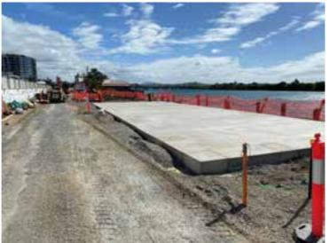
Figure 21: Activity Shelter Slab Complete
