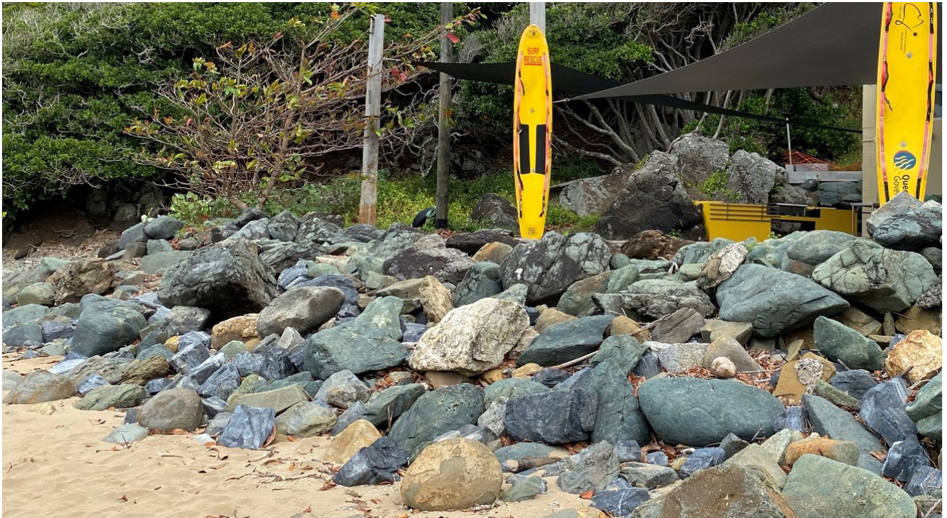
Figure 24: Sarina Beach Surf Lifesaving Club and seawall in front.
