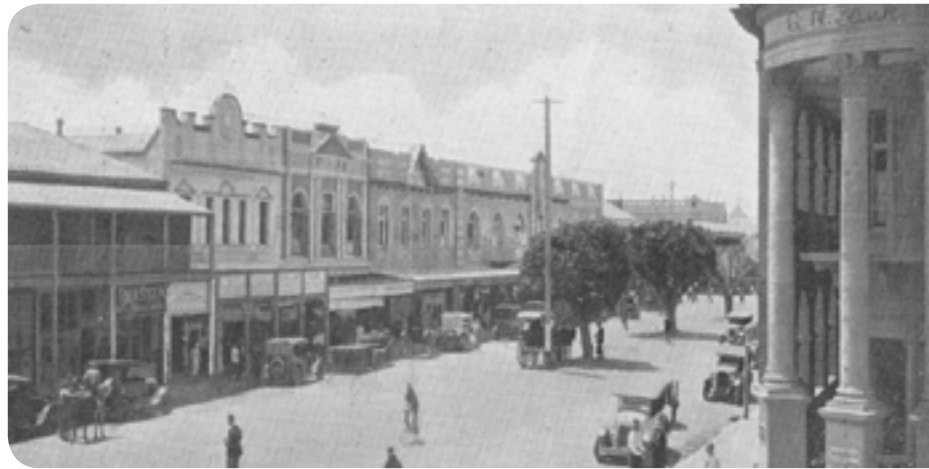
North Side of Victoria Street ca. 1925
