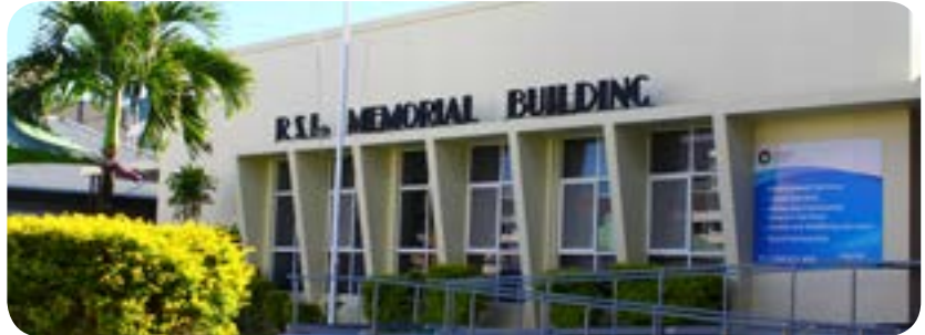
RSL Building, 2016, Mackay Regional Council
