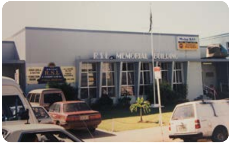
RSL Building 1992, Mackay Regional Council
