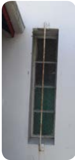
Far Right: Visible brickwork and Right: Original windows 2016, Mackay Regional Council
