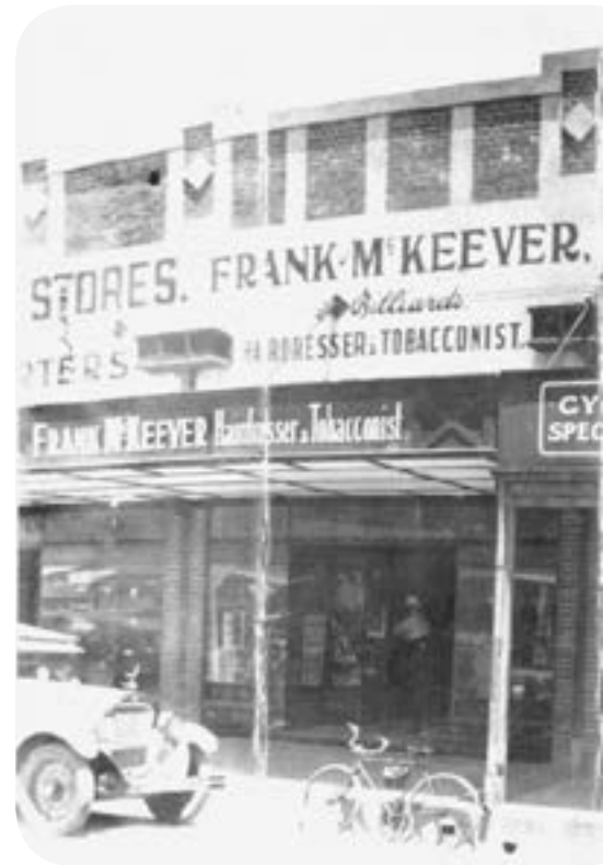
Western side of Sydney Street ca 1920s, Note the original brick detailing on the parapet. Copyright Mackay Regional Council Libraries Image No. qmc 1960
