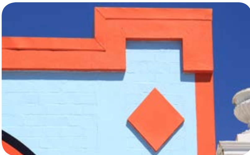
Brickwork detail covered by paint, McKeever's, 2016, Mackay Regional Council
