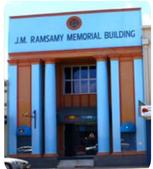
JM Ramsamy Building, 2016, Mackay Regional Council
