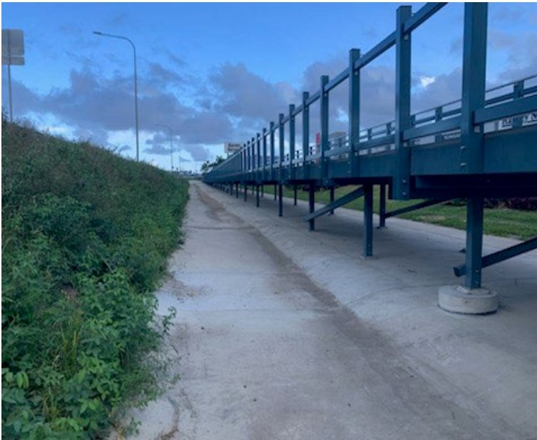
Elevated boardwalk in TMR road reserve
