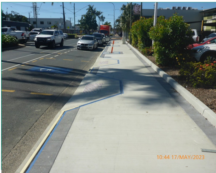
Victoria Street new footpath in front of Dan Murphy's
