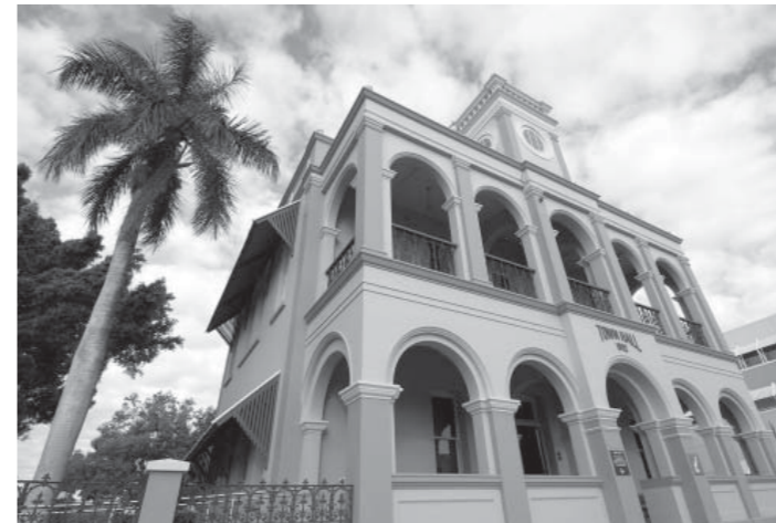
Mackay Town Hall, Sydney Street
