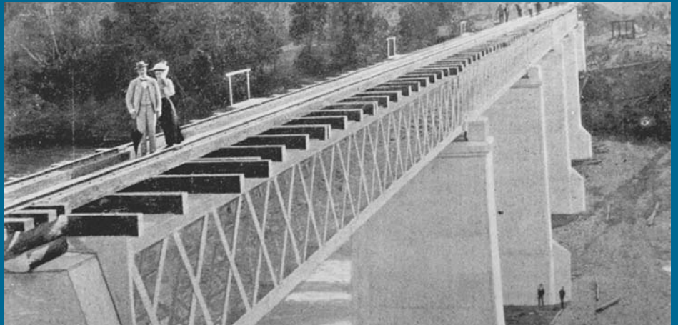
High-level railway bridge at Mirani, ca. 1897.
