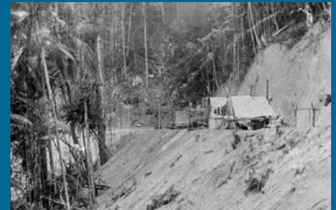
Construction of the road to Eungella, ca 1906-1907.
