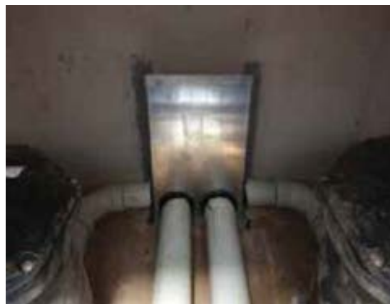
Figure 3 - Typical Outlet Weir Wall
