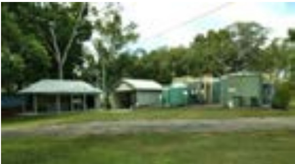
Camp Kitchen, Laundry and Package Treatment Plant located within the Seaforth Camping Reserve.
