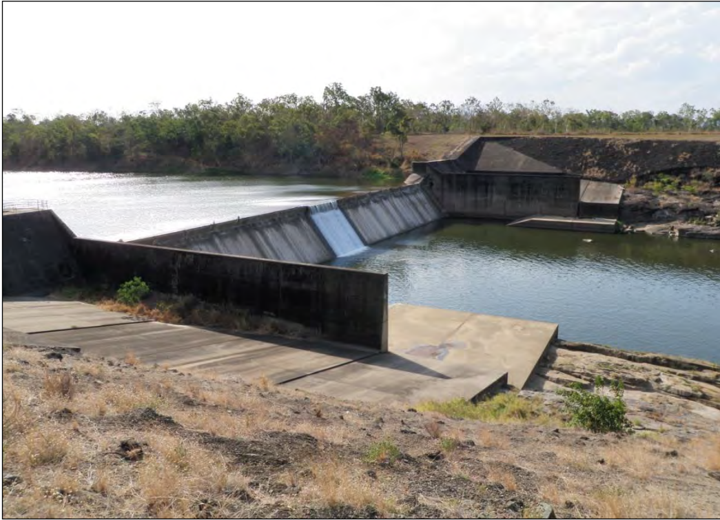
Figure 2.1 - Mirani Weir looking upstream (taken from the right bank)
