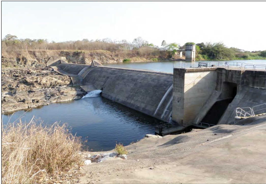
Figure 2.3 - Dumbleton Weir, looking upstream (taken from the left bank)
